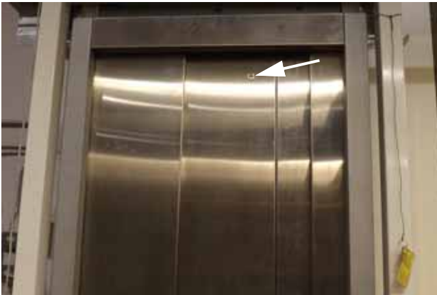
Figure 4: Auto Slim Landing Doors Emergency Opening
